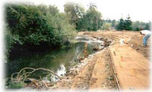
▲ ABOVE, SHOWS FABRIC ENCAPSULATED SOILS LIFTS DURING CONSTRUCTION
