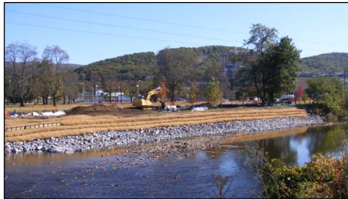
Photograph showing riverbank during placement of the fabric-encapsulated soil lifts.
