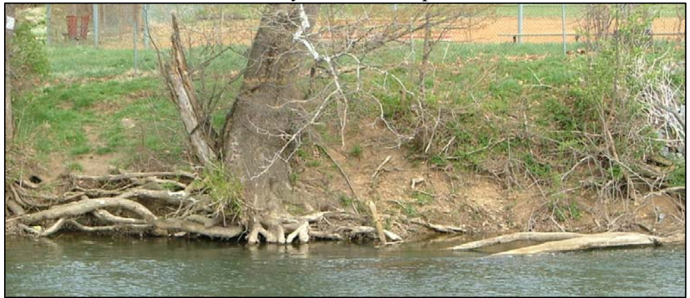
Photograph of a typical eroding bank along the South River.
