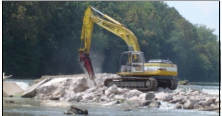
Dam demolition in September 2004.
